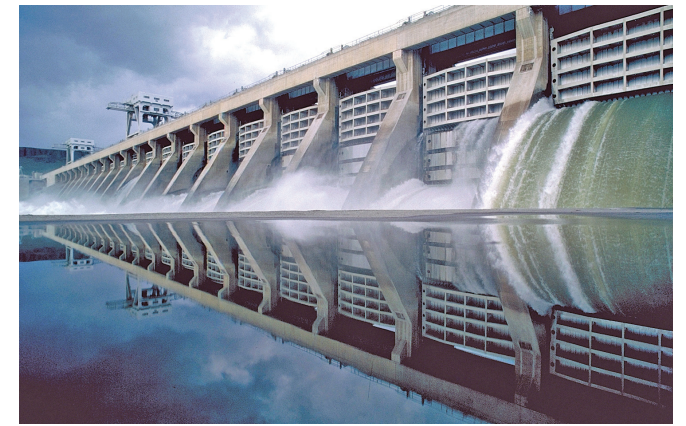
Spill helps juvenile fish pass the dams on their way to the sea.
